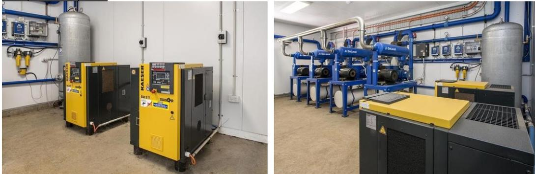
**Caption:** Two Kaeser SX 3 T series rotary screw compressors with integrated refrigeration dryers, complete with air treatment package and air receiver installed at Bannister Downs Dairy Farm.
