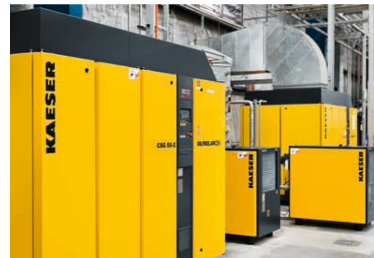
Image left: Central compressed air station in the brewery.
