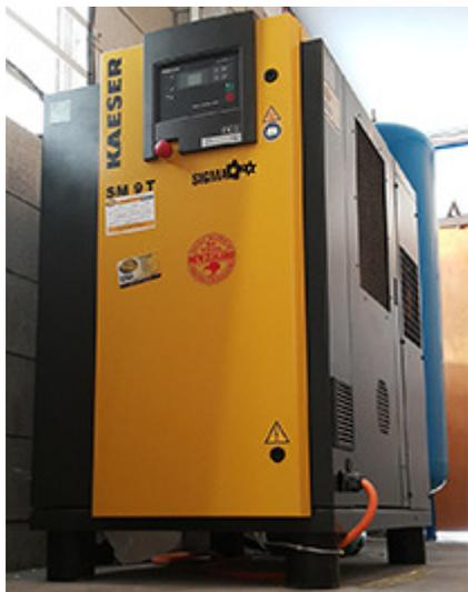
Caption: 3DPrint-AU chose to invest in a Kaeser SM9T series rotary screw compressor with integrated refrigeration dryer, to reliably meet their demand for compressed air.
